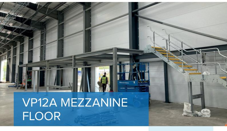
MetStructures were contracted to undertake the design, detailing, fabrication, and erection of 263 tonnes of steelwork as part of an extension to an existing cardboard manufacturing facility owned and operated by **ProGroup Board GmbH.**
