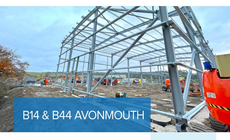
MetStructures were contracted by Barnwood to undertake the design, detailing, fabrication and erection of 301 tonnes of steelwork for two new warehouse units in Avonmouth:
