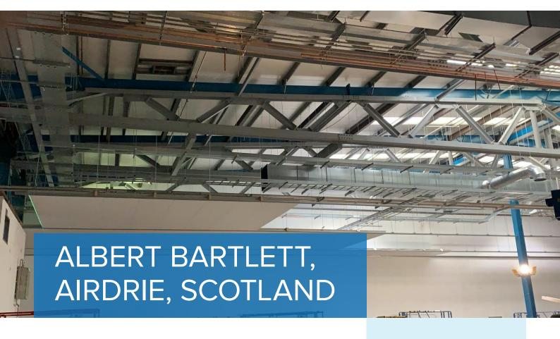
MetStructures were contracted to undertake structural strengthening works to an existing portal framed structure by installing new trusses to the underside of the roof.
