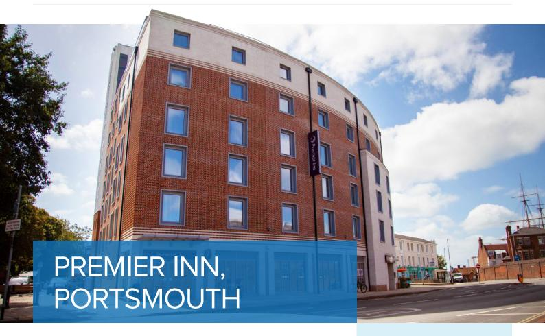
The faceting façade highlights the flexibility of MetStructures Light Gauge Steel Frame solution proving that it's not just for boxes.
