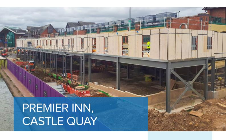
The MetStructures team installed the hot rolled podium and light gauge steel frame with limited access on site with an adjacent canal, multi-story carpark and shopping centre.
