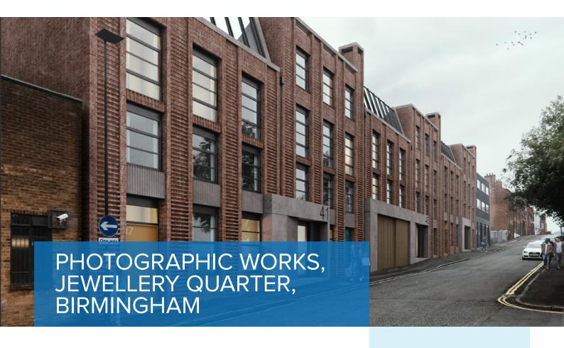
MetStructures are supplying the Hot-Rolled podium and Light Gauge Steel Framing System above for this 4-storey project.
