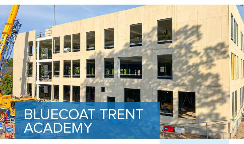
MetStructures were contracted by Bowmer + Kirkland to undertake the design, detailing, fabrication, pre-assembly, and installation of light-gauge pre-assembled panels for a new school being constructed in Nottingham.
